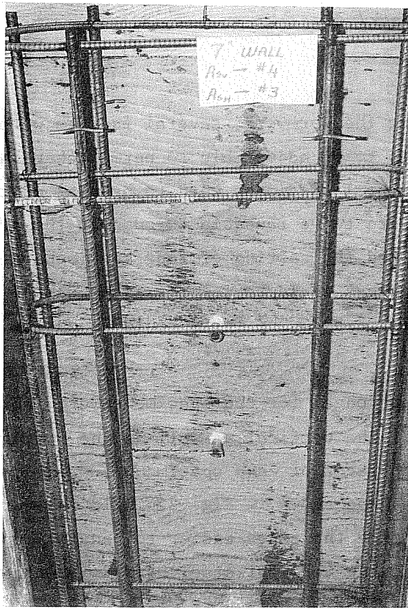
Fig. 2.6 Horizontal "hairpin" reinforcement
